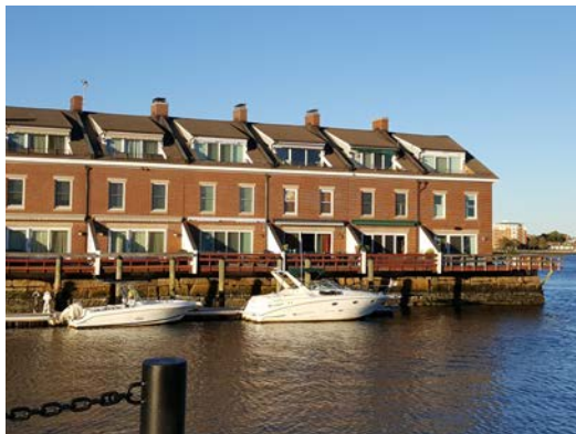
Buildings Overhanging Wall
